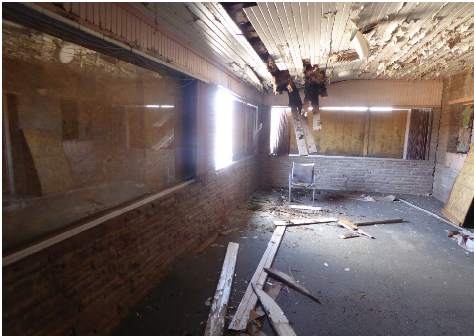
Figure 14. Interior damage including collapsed ceiling.
