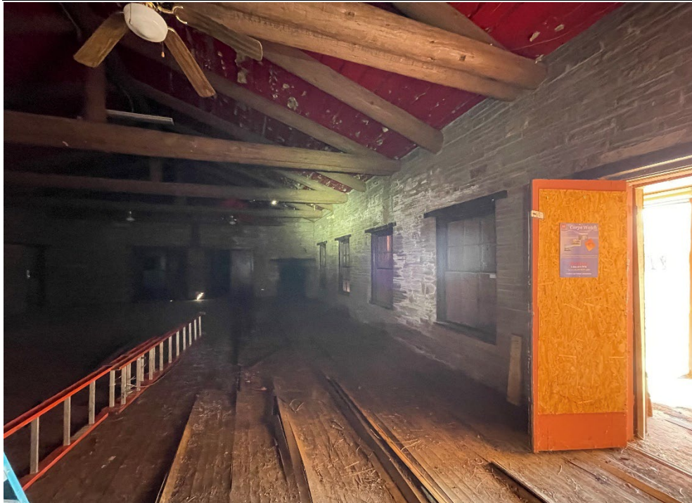
Figure 13. Severe floor and ceiling damage within interior main room of Lodge
